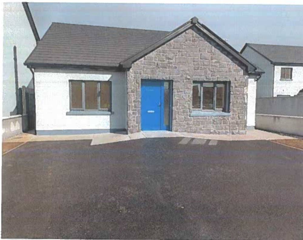
Newly constructed Traveller Specific Accommodation in Athenry
