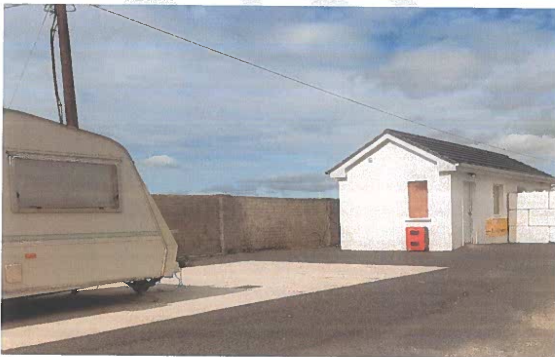
Halting site bay with caravan and welfare unit in Capira Halting Site, Portumna
